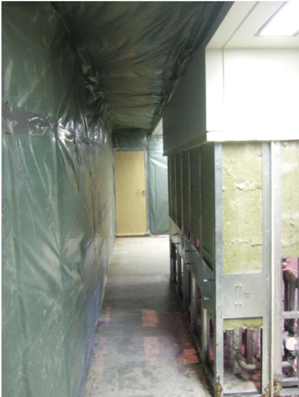
Figure 2: Dust protection – view from renovation area
